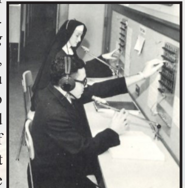
Sr. Chiara helping out with the switchboard
